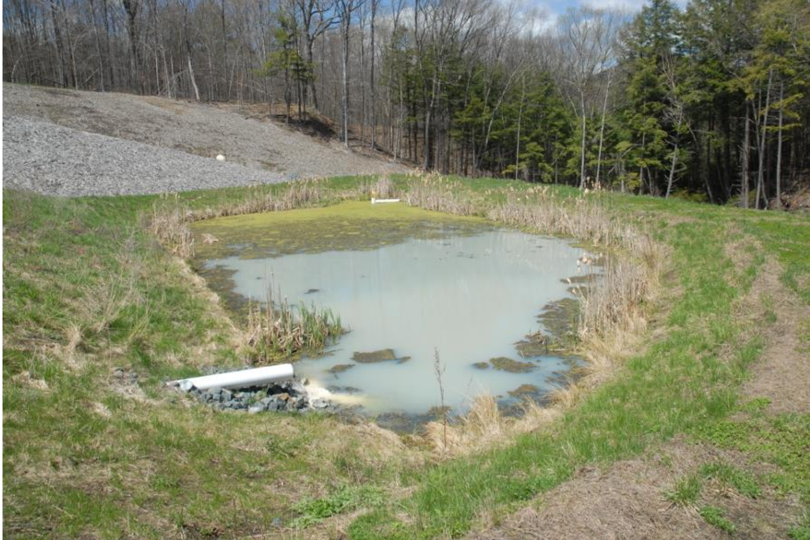
30. Passive Treatment System looking northwest showing secondary wetland (Milestone Heritage Consulting, May 2021).
