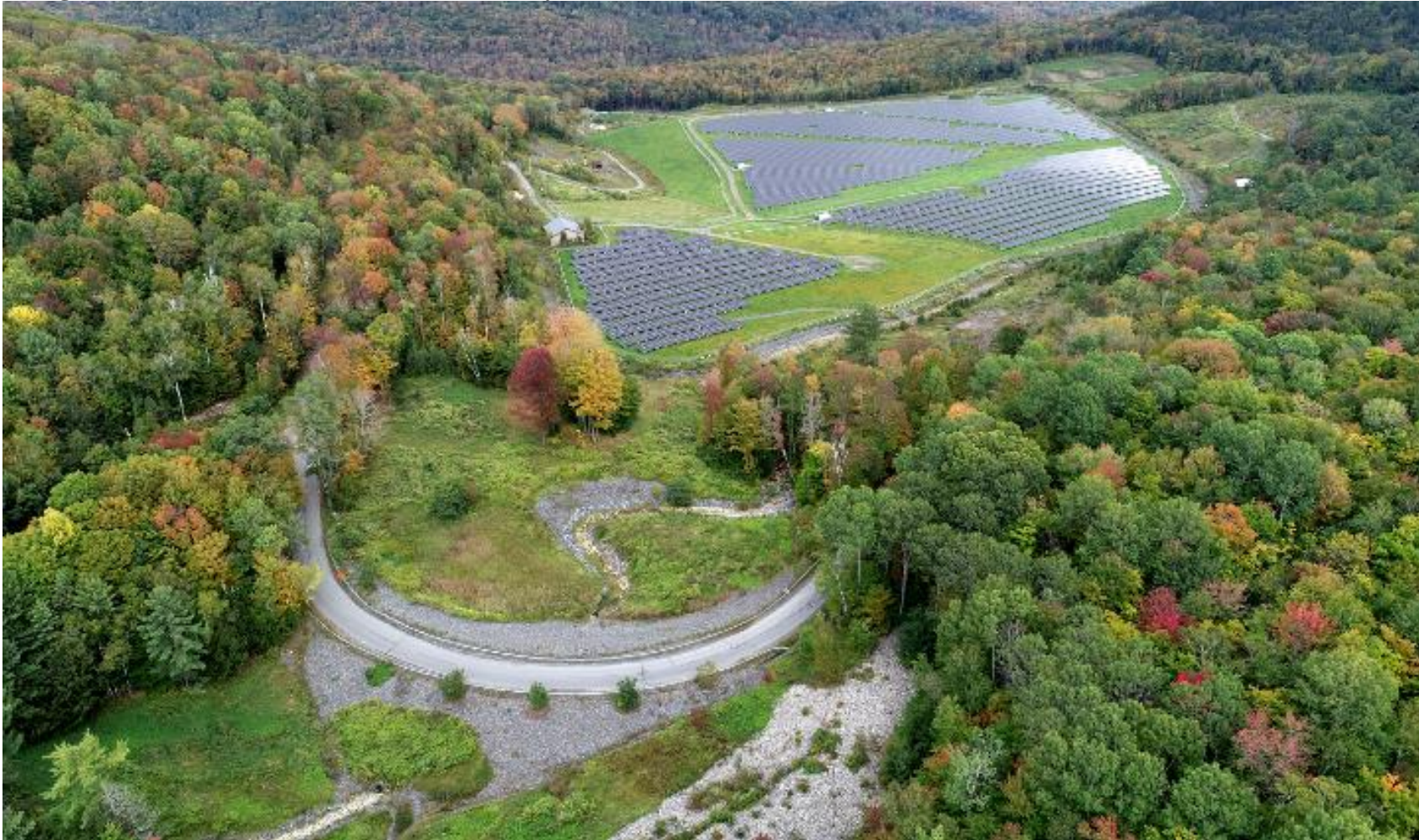
31. Aerial view of Solar Electric Panel Array looking northeast (Doucet Survey, September 2021).
