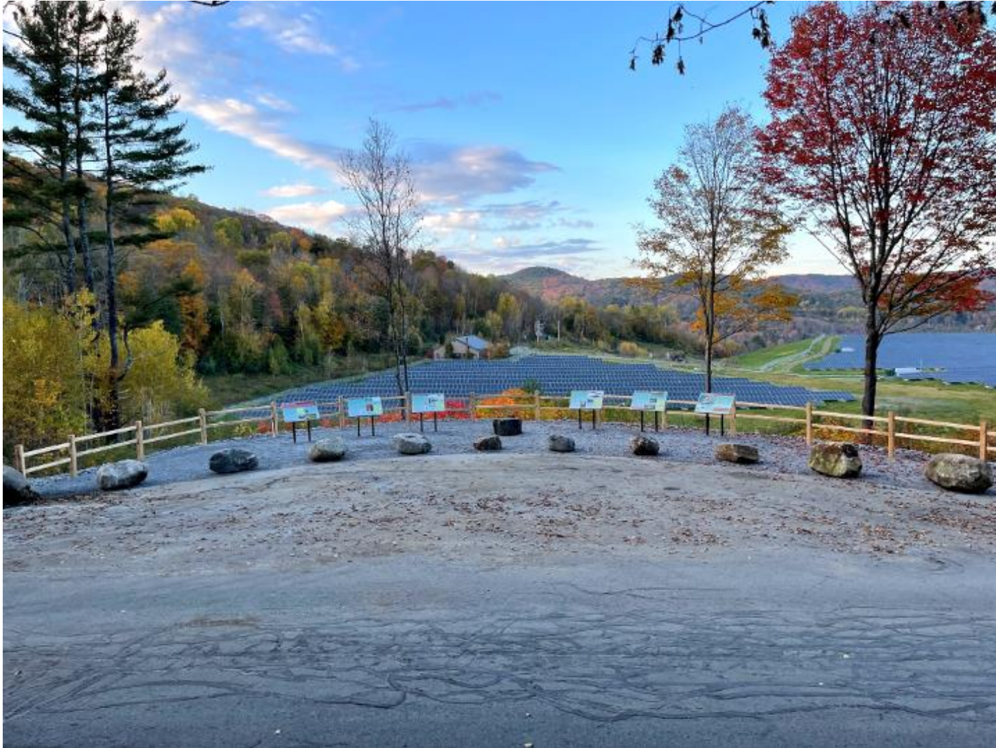
45. Mine Road Bus Turnaround (TP-1-2/Solar Array Overlook) Installation looking north (Nobis Group, October 2021).
