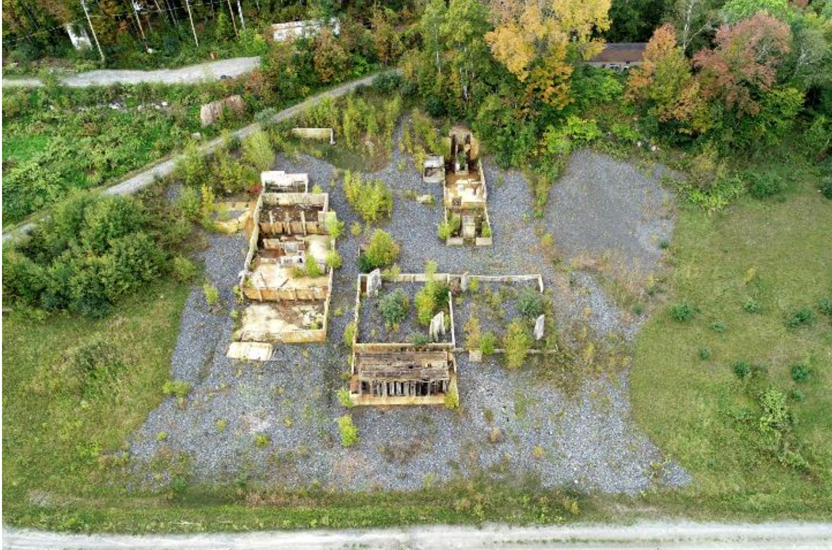
57. Aerial view of World War II Flotation Mill looking west (Doucet Survey, September 2021).
