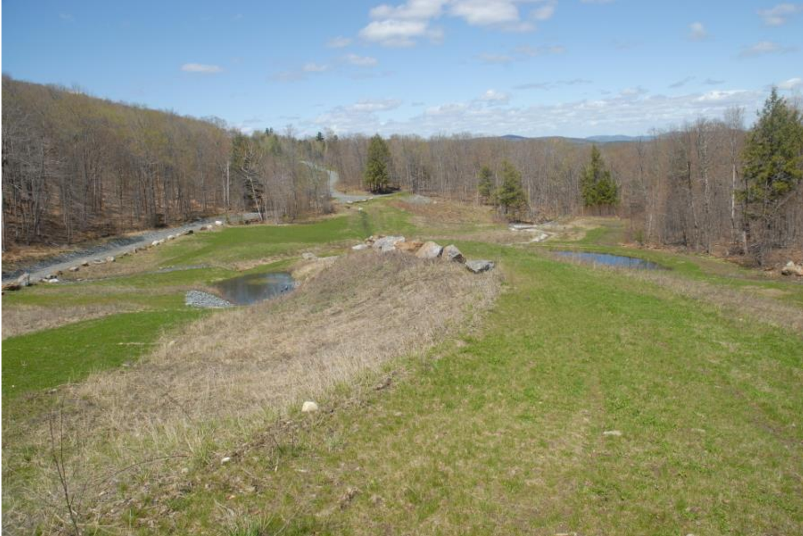
6. South Mine area looking north (Milestone Heritage Consulting, May 2021).
