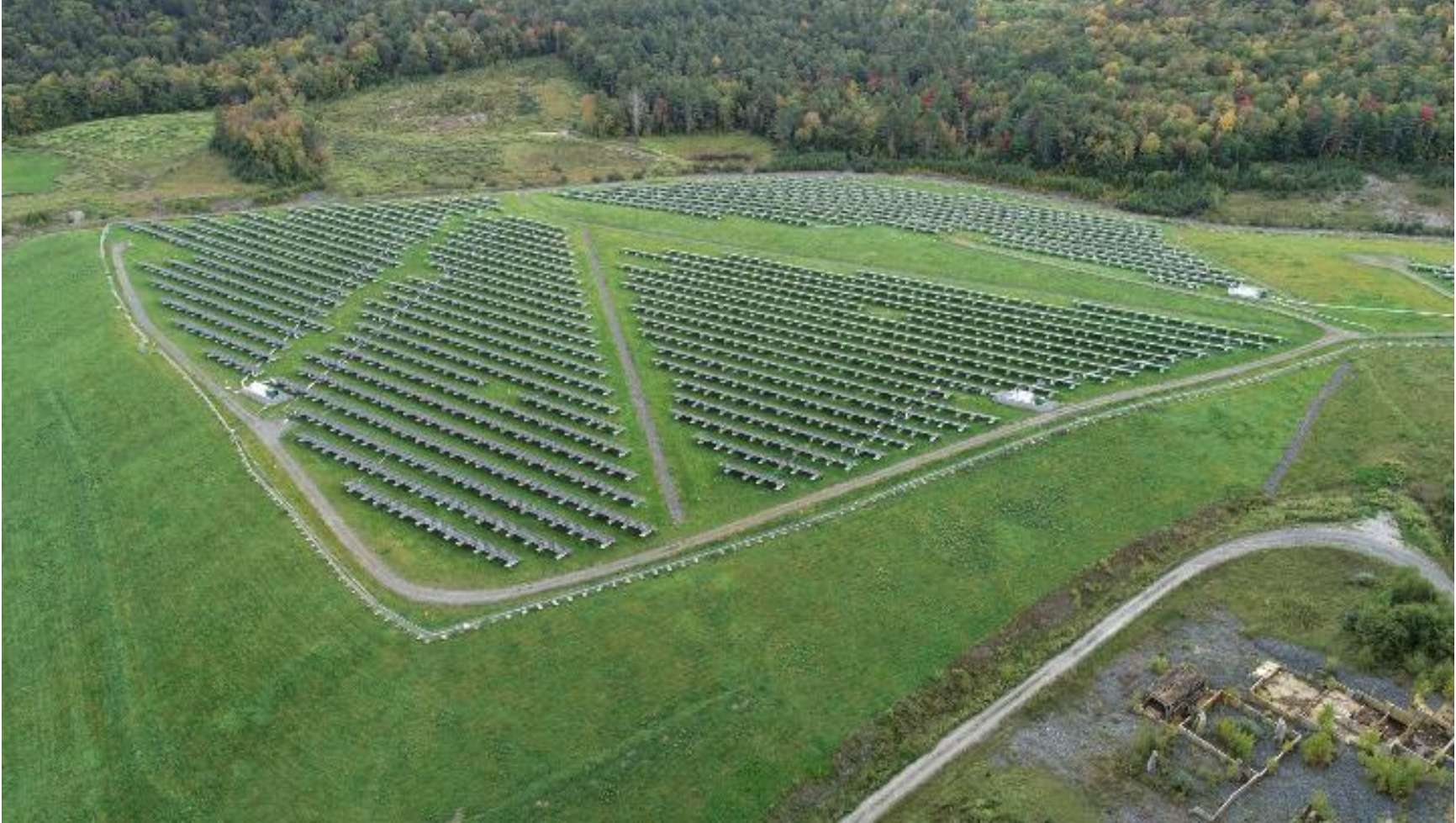
35. Aerial view of Solar Electric Panel Array looking southeast (Doucet Survey, September 2021).
