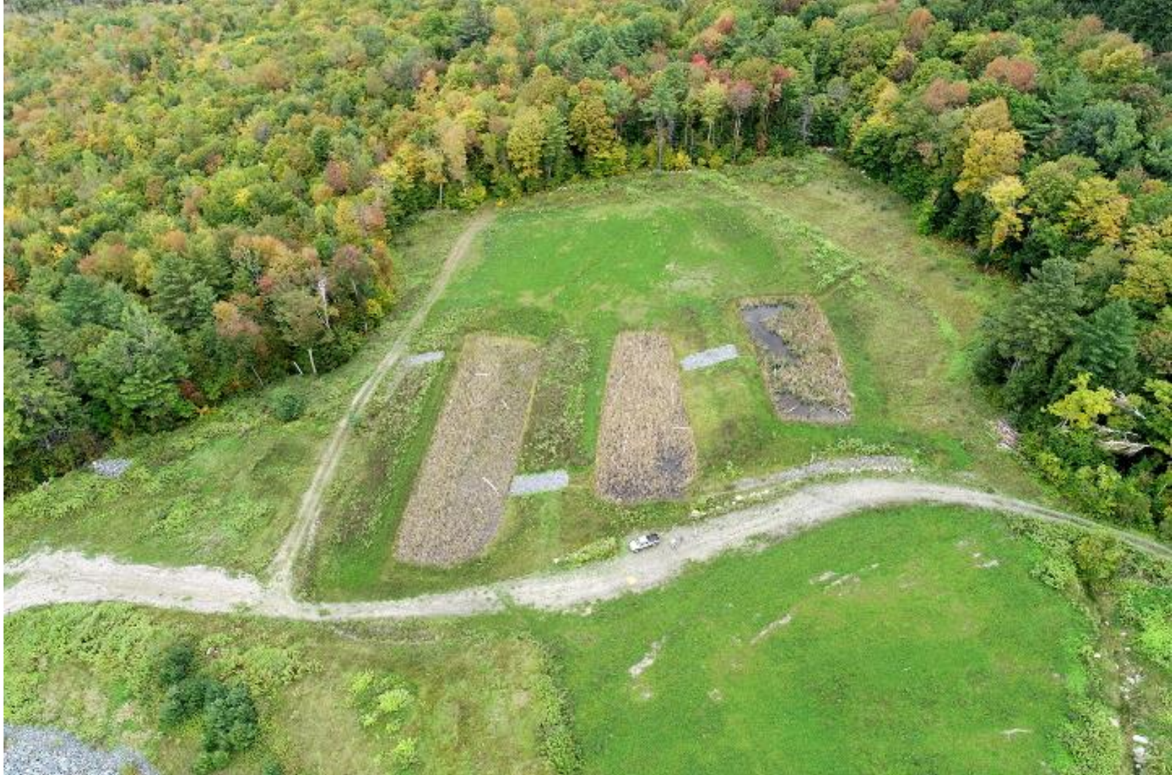
41. Aerial view of reclaimed Borrow Area constructed wetlands looking northeast (Doucet Survey, September 2021).
