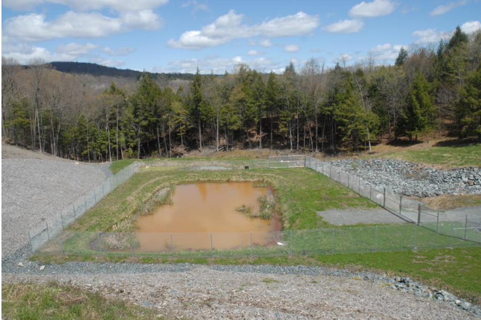
29. Passive Treatment System looking north showing vertical flow pond (Milestone Heritage Consulting, May 2021).
