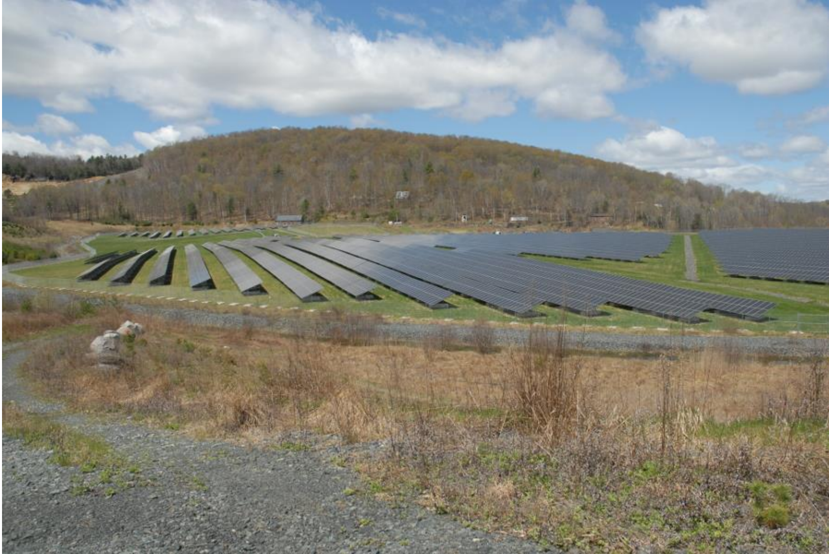
38. Solar Electric Panel Array looking northwest (Milestone Heritage Consulting, May 2021).
