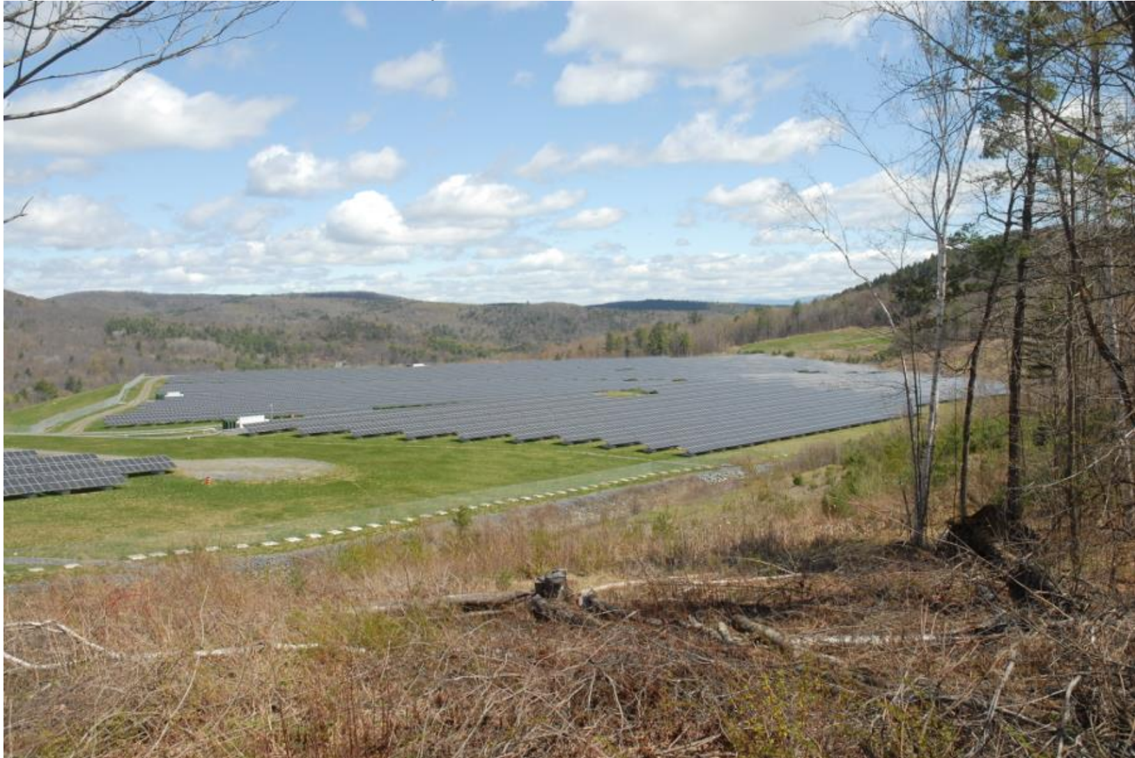
37. Solar Electric Panel Array looking northeast from Mine Road bus turnaround (Milestone Heritage Consulting, May 2021).
