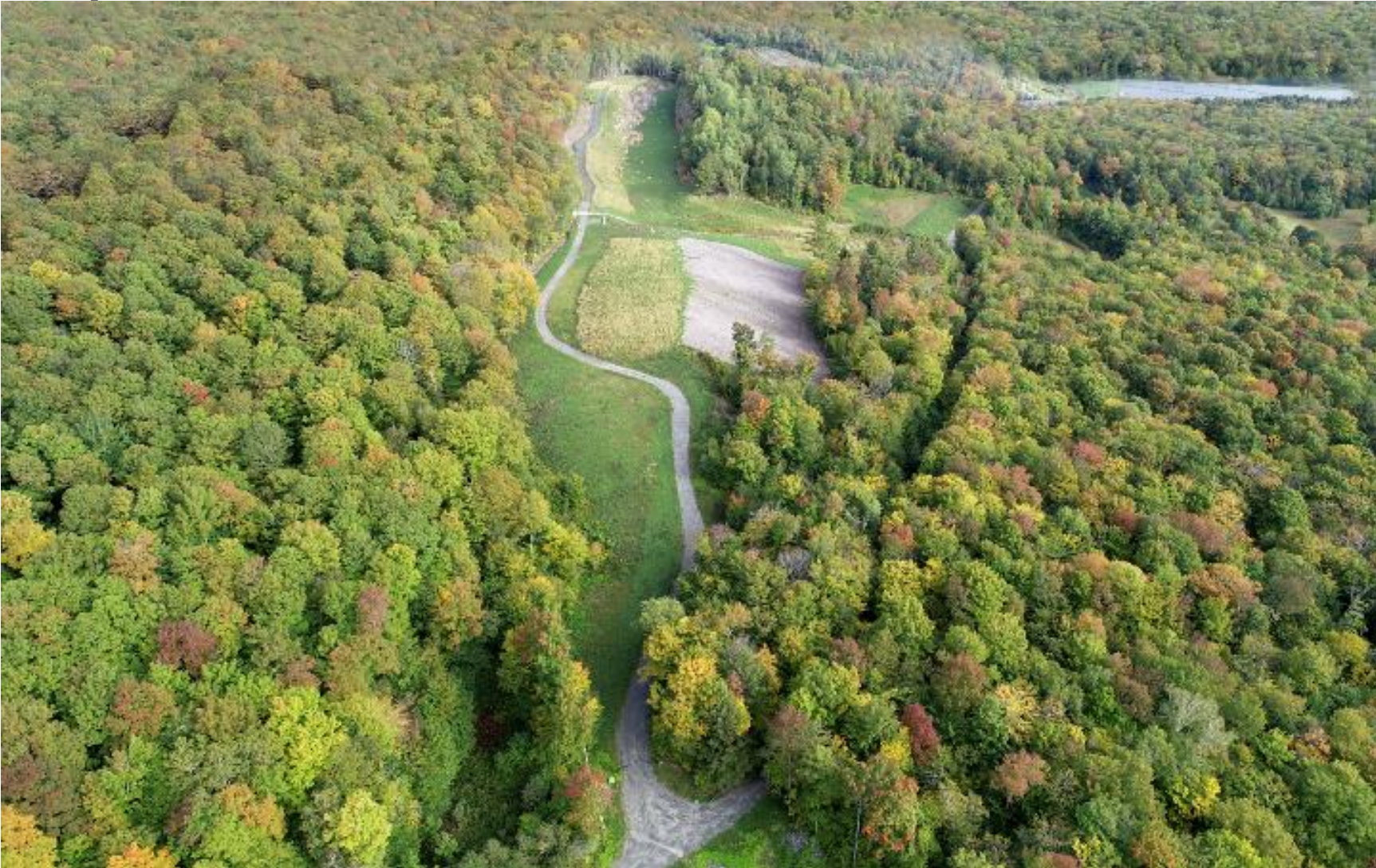
9. Aerial view of reclaimed South Open Cut looking north (Doucet Survey, September 2021).
